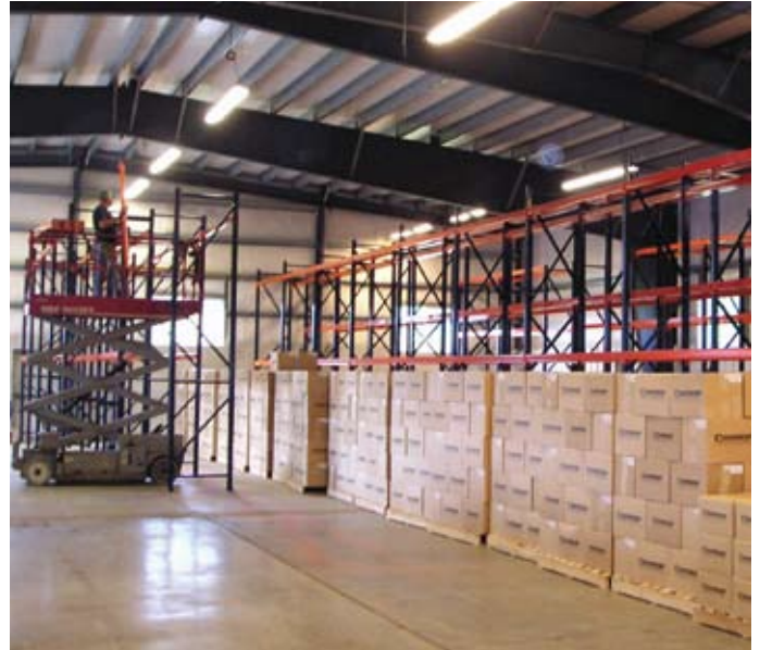
Racking being assembled in Conewango's new warehouse.
