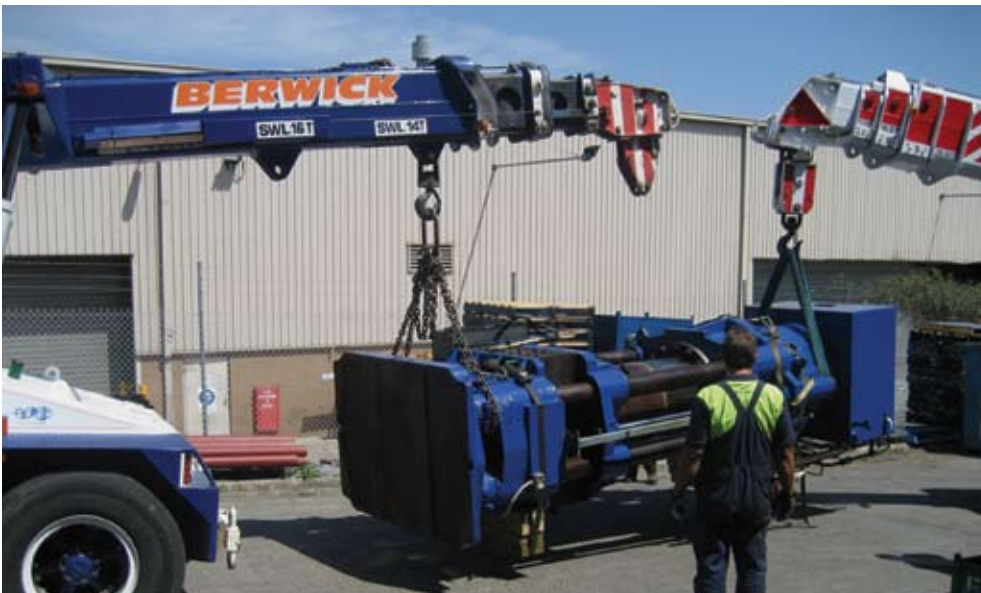
Lifting the 24.5 tonne press which hadn't moved for the last 25 years.
